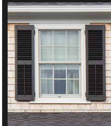
Traditional wood-louver shutters and hardware were purchased from New England Shutter Mills in Lawrence, Mass.
