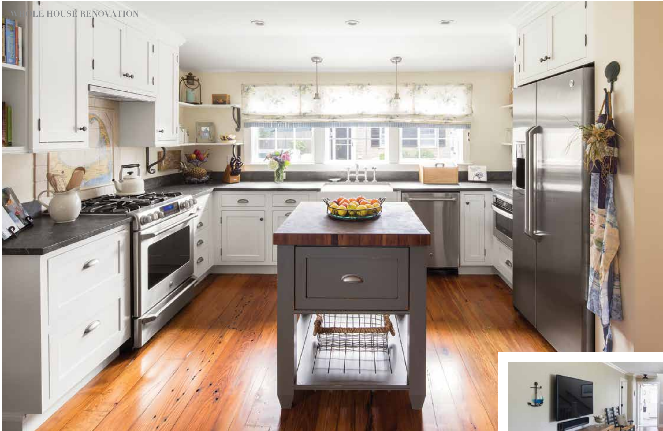
Left: The kitchen was expanded using space taken from a half bath.
